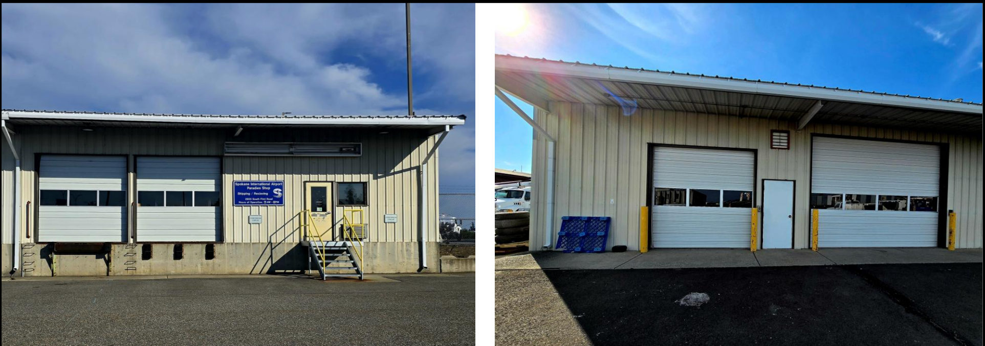
Air Cargo Exterior – Front Loading Dock & Service Counter Entrance, Back Loading Dock
