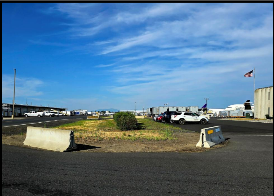
Parking Lot Expansion
